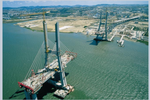
Vasco da Gama Brücke, Portugal
