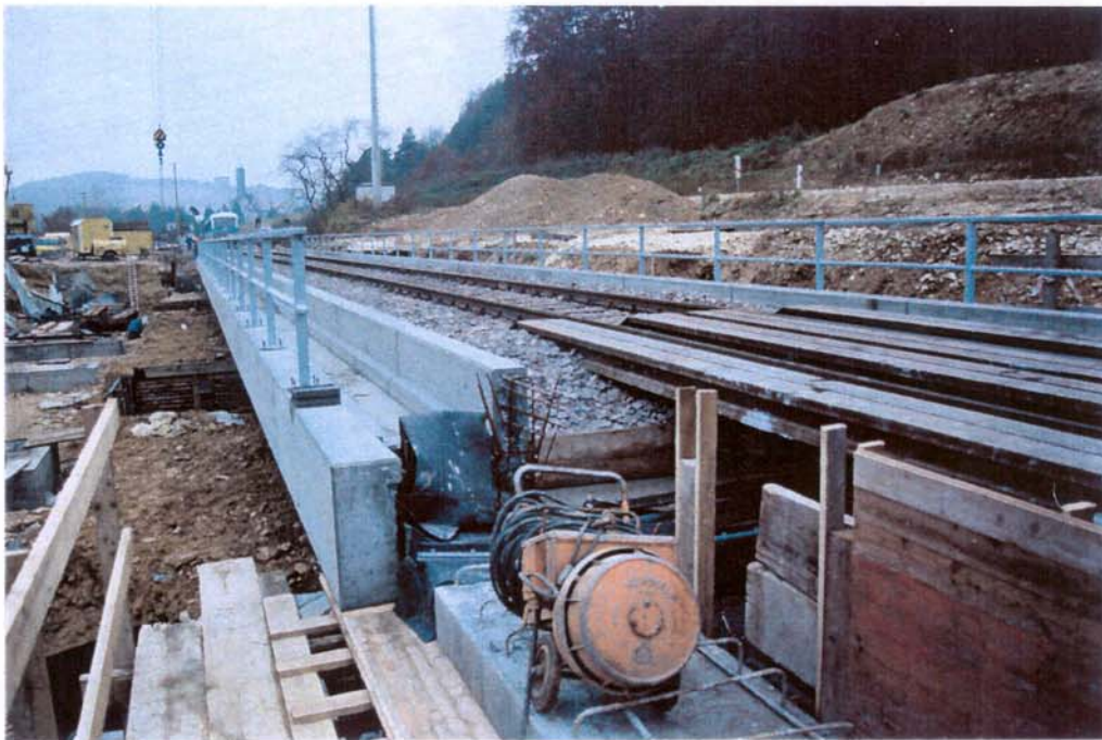
General view of the bridge
