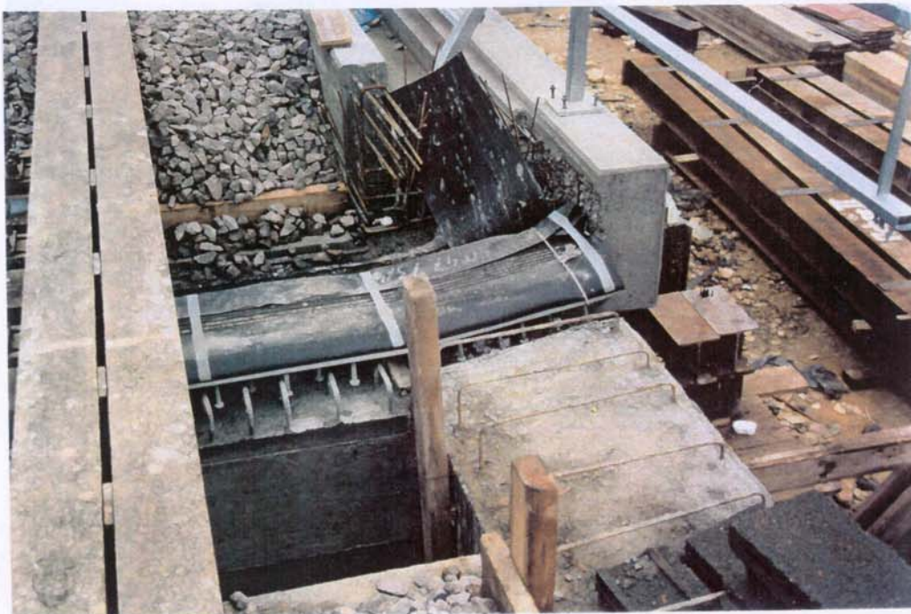
Fully assembled expansion joint type DB 130 placed into the recess
