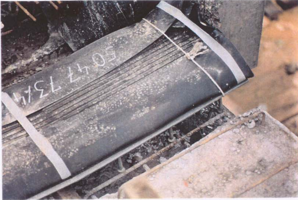
Detailansicht Dehnfugenendabschluß Detail view edge plate of the expansion joint
